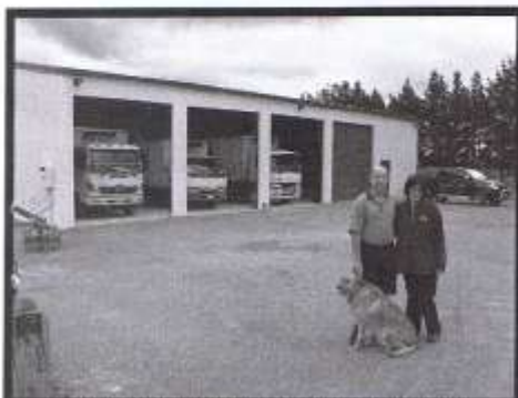
Adjusting the bay widths on this shed used by a food distribution business reduced waste space between the trucks and increased valuable storage space.
